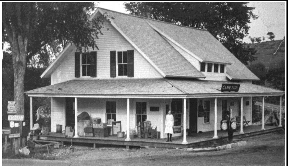
Photo (above): Charles Wheaton built this store across from his family home sometime between 1900 and 1920. He had worked for his father, Simeon, in the general store that once stood across from the Wheaton home at the foot of Providence Pike. Simeon died in 1917 and we believe his store was destroyed by fire. Photo (right): Meier's store after Hurricane 1938. Photo Page 1: The date of this photo is unknown, but we believe the store was then owned by Joseph and Anna Meier. They lived above the store where they raised their three children Joseph, Charles, and Anne. The aroma of the evening meal would often greet you as you entered the store. The family could be seen sitting around the kitchen table as Mrs. Meier got up to wait on you. Please submit your personal remembrances of Meier's Store and the Meier Family to ehsarchives@gmail.com . The Eastford Historical Society would greatly appreciate your support. We always welcome new members and/or contributions toward our efforts to preserve Eastford history. We are also very grateful to those of you who have continued your support either through member and/or donation to: Eastford Historical Society, P.O. Box 350, Eastford, CT 06242
